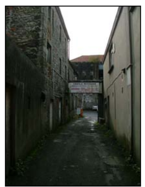
41. Existing vehicular access off Castle Street
